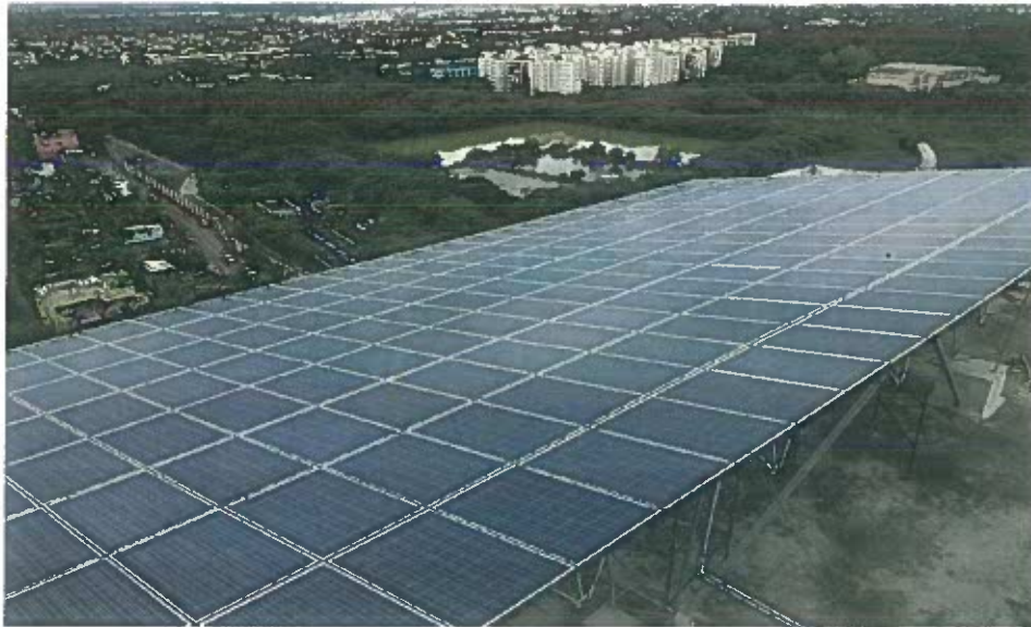
1 MW rooftop Solar PV for a leading glass solutions company at Chennai
