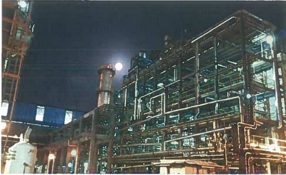
First of a Kind LSHS (low sulphur heavy stock) firing in HRSGs at a petrochemical company. This is amongst the first few Heavy Oil fired HRSGs in the world
