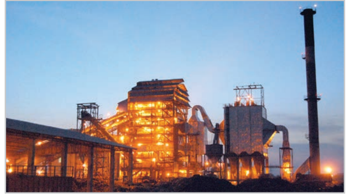
Biomass IPP, 1 X 400 TPD RDF cofired unit
