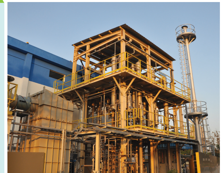
ZLD plant installation at the customer site
