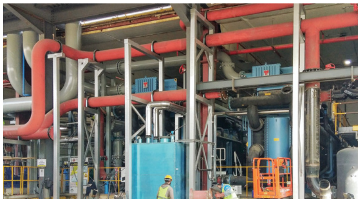
Thermax's vapour absorption chillers
