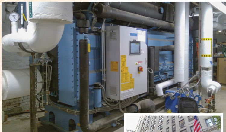
Customised chillers installed at the Hotel.
