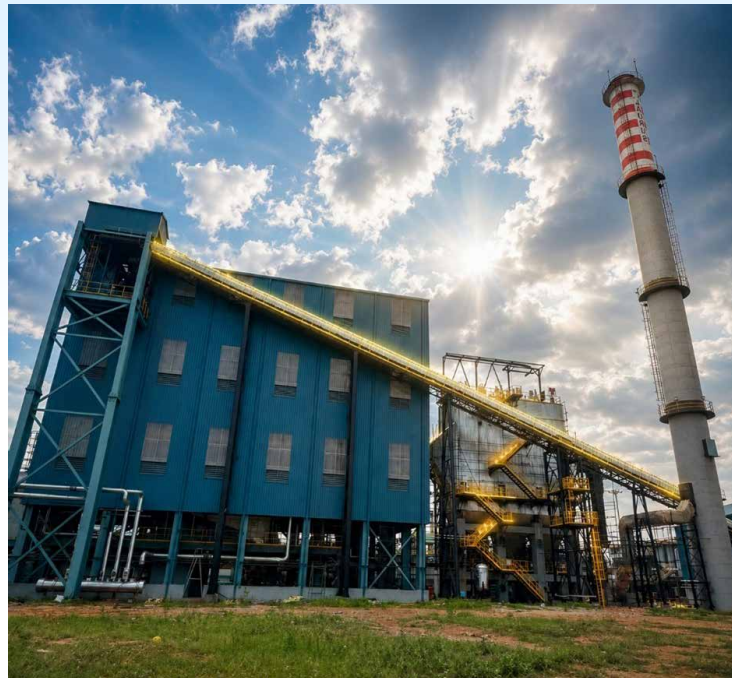
The 27.5 TPH biomass based facility at Laurus Labs in Visakhapatnam
