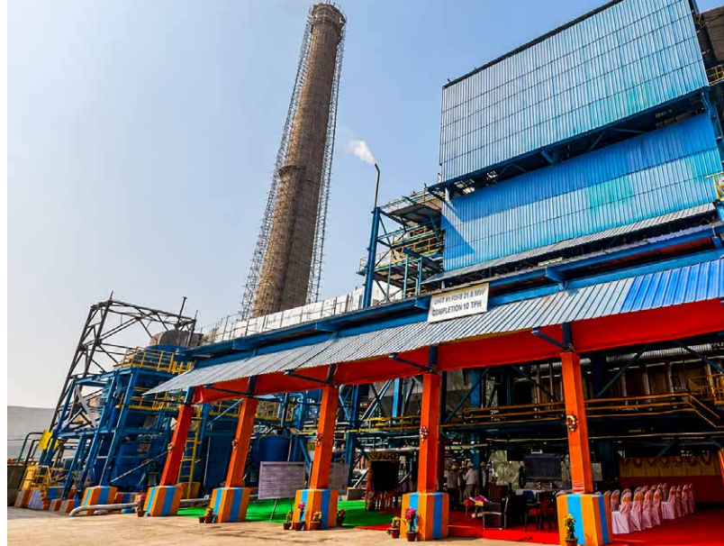
The redesigned dual-fuel boiler erected at the plant
