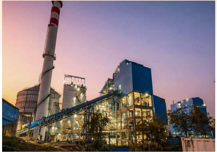
The 5.3 MW cogeneration power plant at Karnataka
