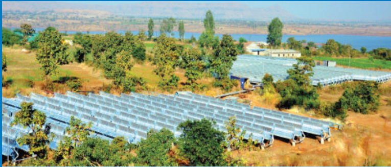
SolPac™ P60 Solar Concentrators for 256KW Solar Biomass Hybrid Distributed Power Generation Plant near Pune
