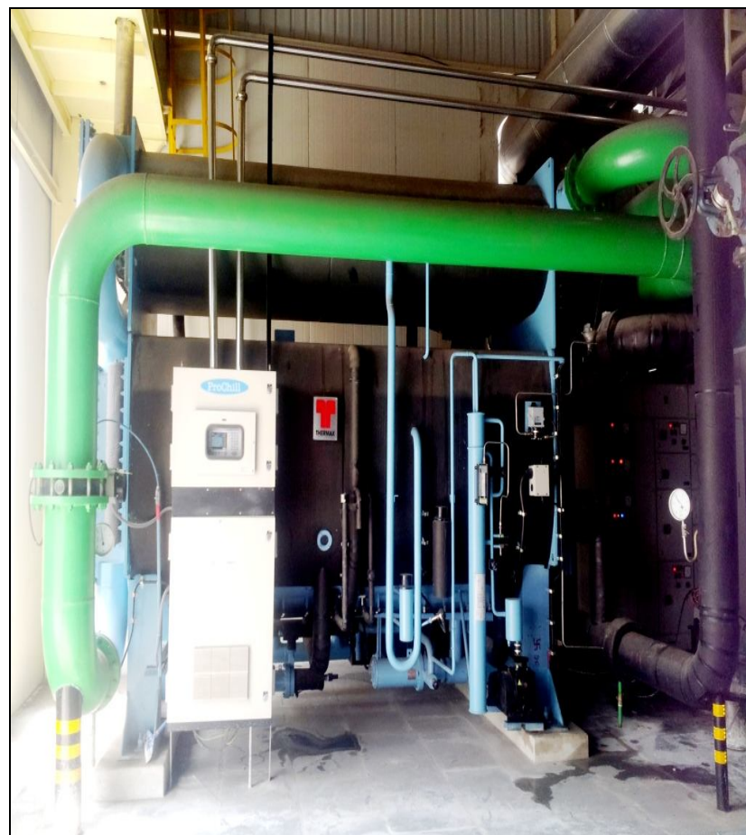
Low Pressure Vapour Chillers in Potato Frying Application
