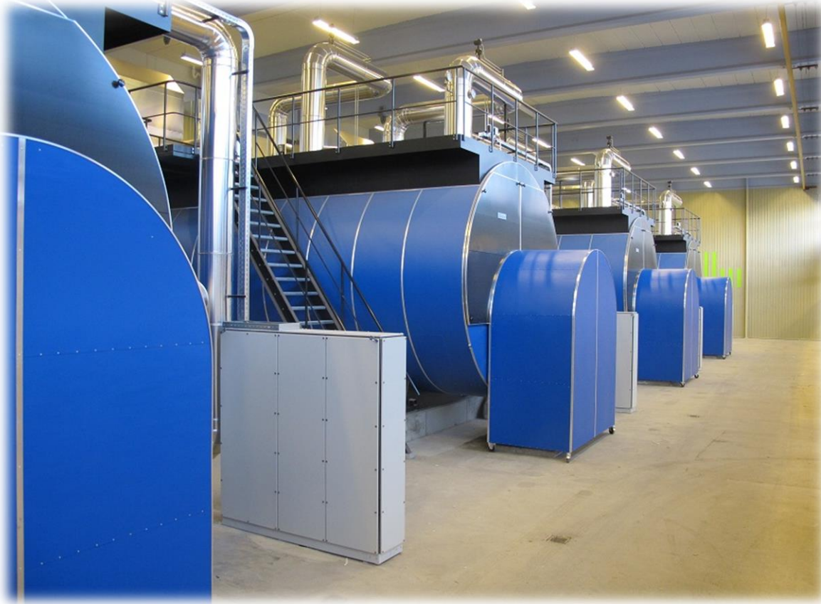
Gas fired boilers for District Heating
