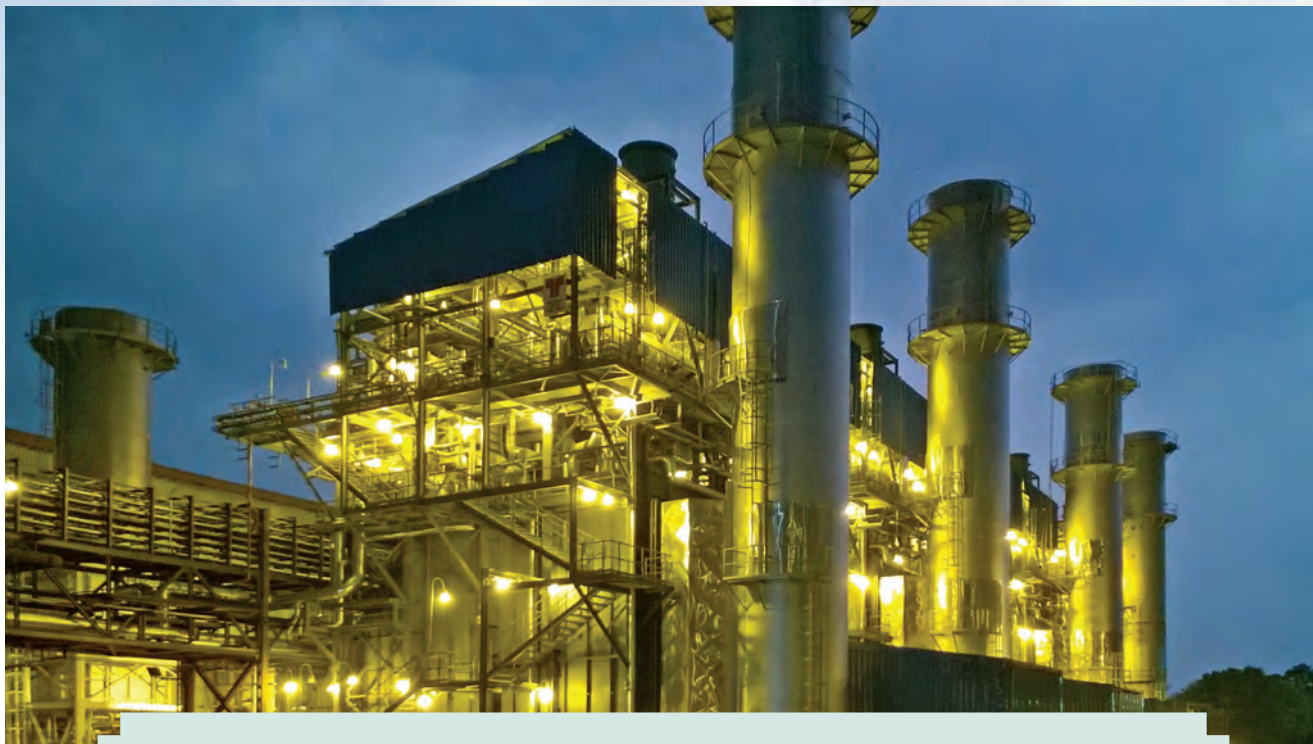
Heat recovery steam generators installed for conversion of an open cycle power plant to a combined cycle power plant in Tripura. Four such dual pressure unfired HRSGs generate 45 TPH hi-pressure and 11 TPH low pressure steam.
