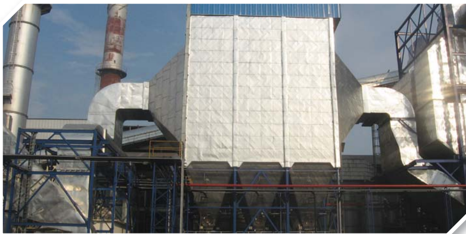
Thermax commissions the sixth Electrostatic Precipitator for Asia's leading sugar and bio-energy producer in Thailand. The ESP handles a gas volume of 4,89,000 m 3 /day.
