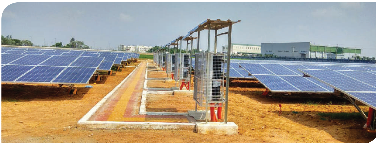
Thermax commissioned a 1.285 MW ground mounted solar photovoltaic system for a leading consumer brand's manufacturing facility at Sri City, Andhra Pradesh. The system is integrated with diesel generator sets to minimise the customer's fuel consumption and dependence on grid power.
