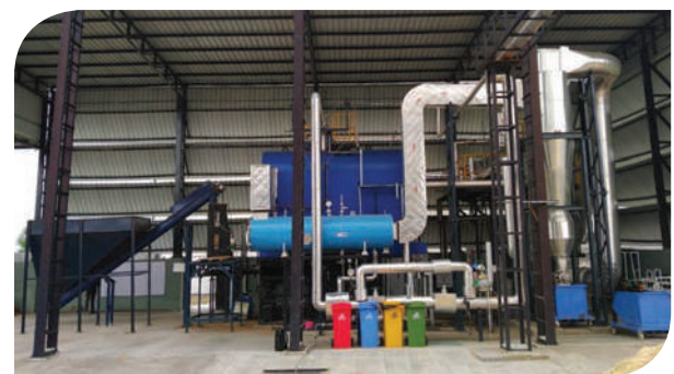
Combloc UFS 30, a 3 TPH boiler installed in Maharashtra for a German multinational producing animal feed. This biomass fuel-based boiler is semi-automatic, designed for small-sized plants.
