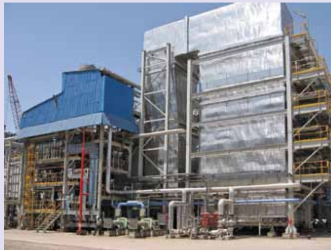
Conversion of equipment for fuel flexibility: ambitious assignment
