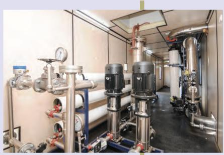
The compact plants are installed in refurbished and air-conditioned 40 feet shipping containers made of stainless steel. They comprise UF membranes, RO pressure tubes and pumps, pressure control devices and transmitters. The ultrafiltration and reverse osmosis systems are linked by PLC to run individually or in tandem.
