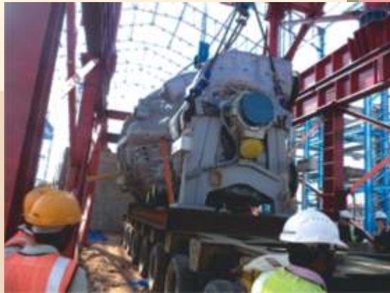
Thermax team installing the steam turbine : proven experience
