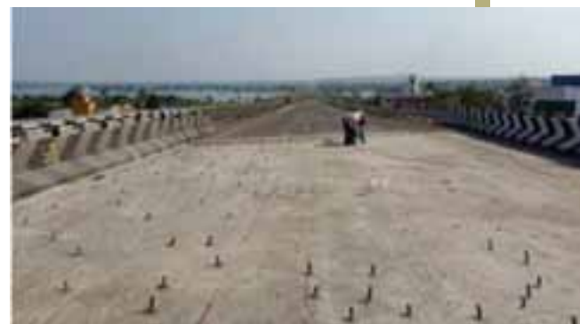
Expressway work in progress: turnkey solution
