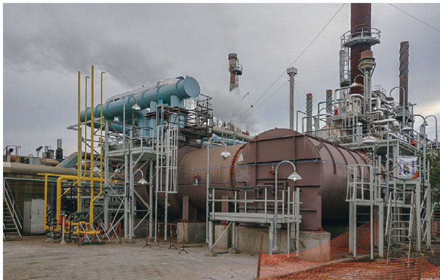
Natural gas-cum-tail gas (CO) fired combustor installed; expanding global footprint - first project in Argentina
