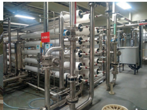
Inside view - filtration unit and (inset) reverse osmosis plant: a reference installation
