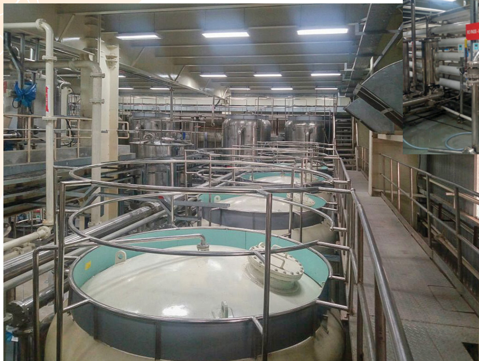
Inside view - filtration unit and (inset) reverse osmosis plant: a reference installation
