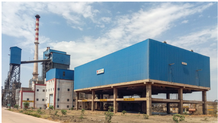
An installed condenser: helping cement plants to be resource productive.
