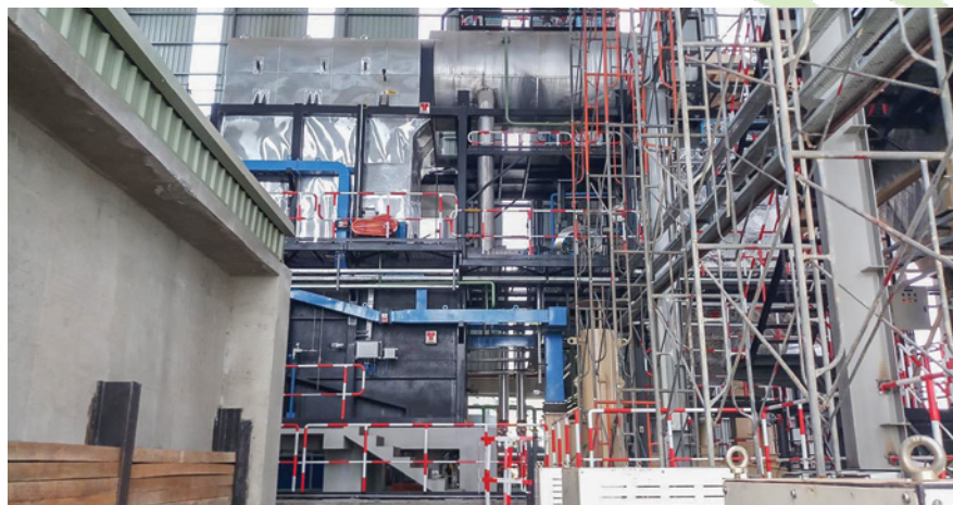
12 TPH Combipac boiler with a reciprocating grate combustor commissioned on a turnkey basis
