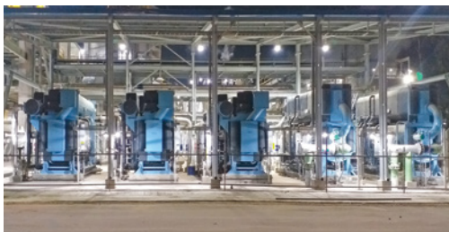
Chillers at CFCL to improve the turbine efficiency
