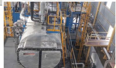
Combipac boiler installation at United Breweries in Rajasthan
