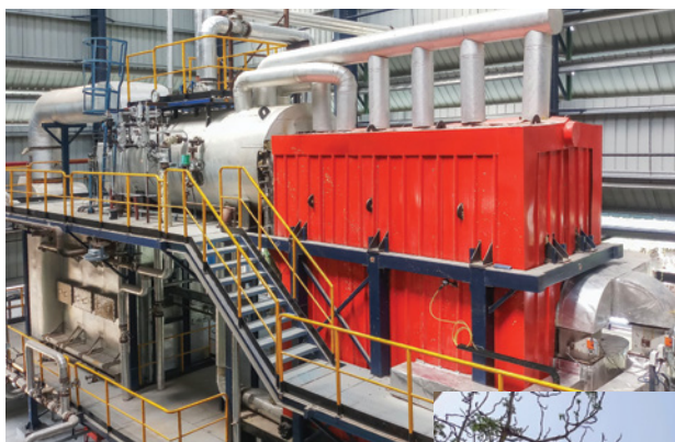
10-ton biomass-fired boiler installed at Malladi Drugs & Pharmaceuticals Limited
