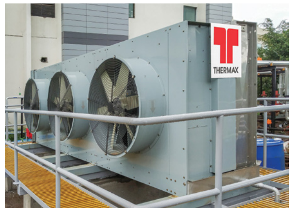
Thermax's adiabatic cooler at a leading data centre company in Pune, maintaining the critical ambient temperature of their server rooms
