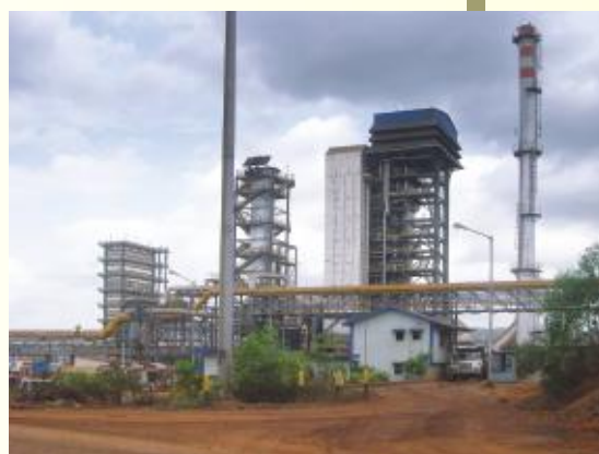
Thermax boiler in action: impressive energy savings
