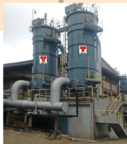
Removing tar from coke oven gas: stringent emission norms
