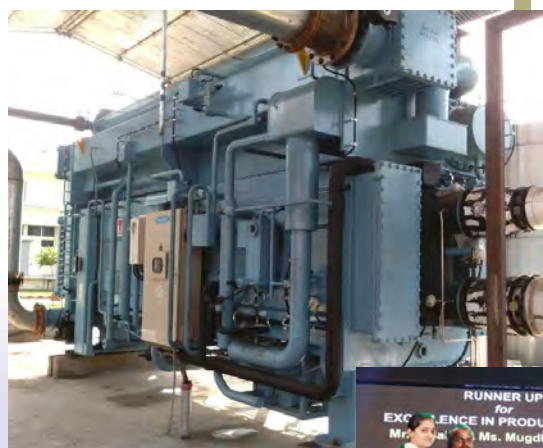
Glycol-free 396 TR chiller for 1°C water at Umang Dairy in Uttar Pradesh, and (right) Thermax's Mugdha Kulkarni and P. Babu accepting the award at the 10th Bry Air Awards
