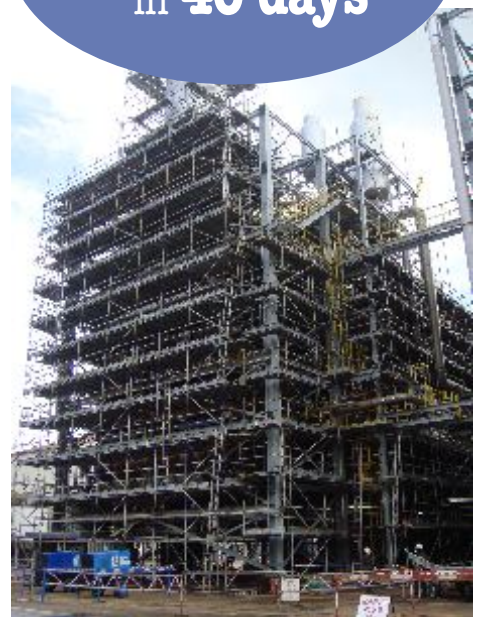
Boiler retrofit in Malaysia: enhancing efficiency
