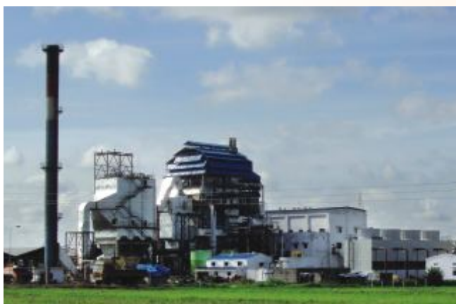
Thermax installation at Shalivahana: power from municipal waste
