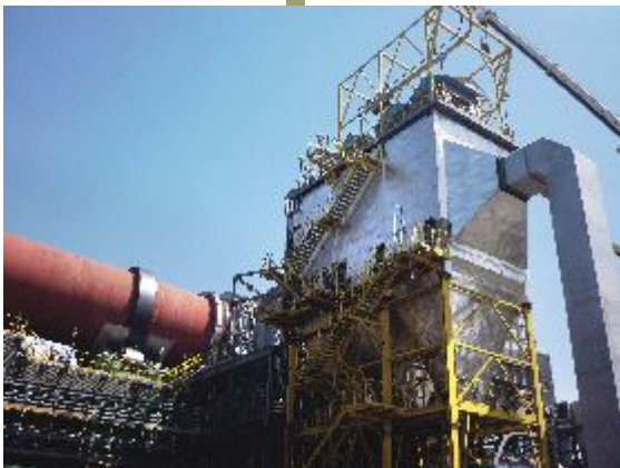
Air pollution control systems : implementing complex projects
