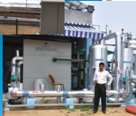
The solar collectors and (below) triple effect chiller : Indigenous R&D
