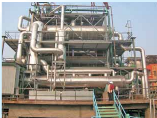
Thermax boiler for sugar industry : Thai installation
