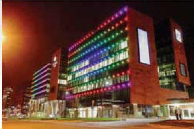
This commercial complex in Zagreb, Croatia's capital, is air conditioned by a Thermax chiller
