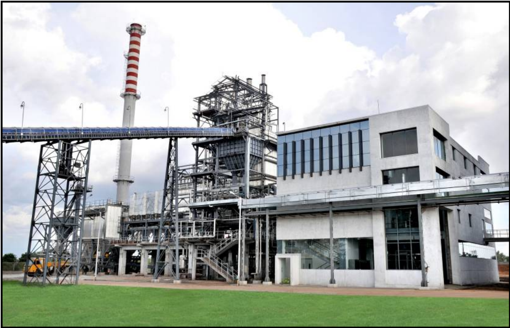
Spent-wash fired boiler at a distillery
