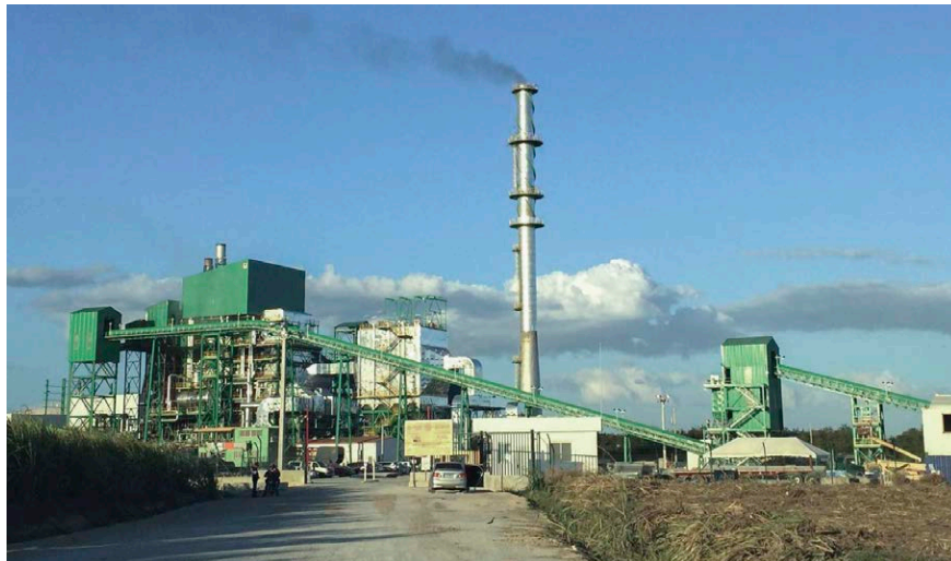
The 140 TPH travelling grate boiler generates 30 MW power
