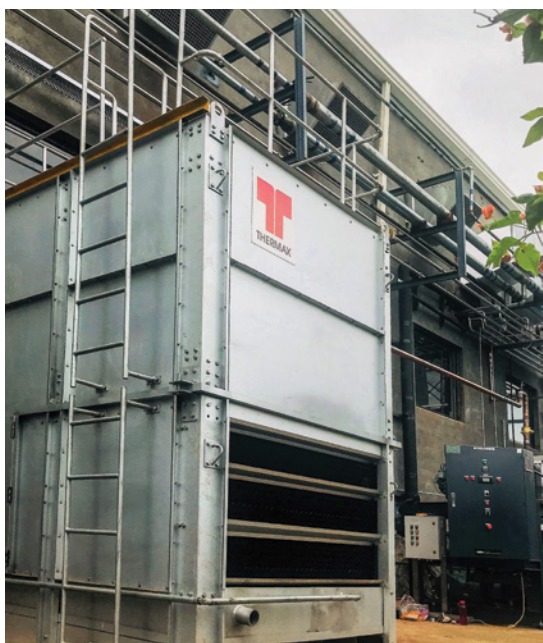
80 TR evaporative condenser installed at the customer site
