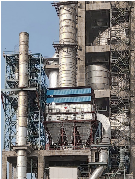
Installation of a bag house
