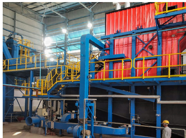
8 ton biomass boiler supplying 'green' steam
