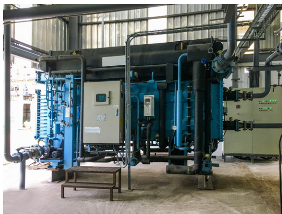
360 TR capacity vapour absorption chiller
