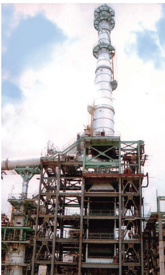
1 unit of 13.5 TPH, 30.5 kg/cm 2 g, 280°C, out board steam generator on cracking furnace
