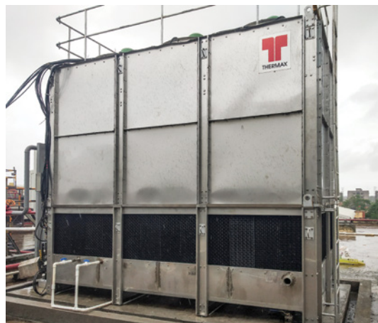
300 TR evaporative condenser
