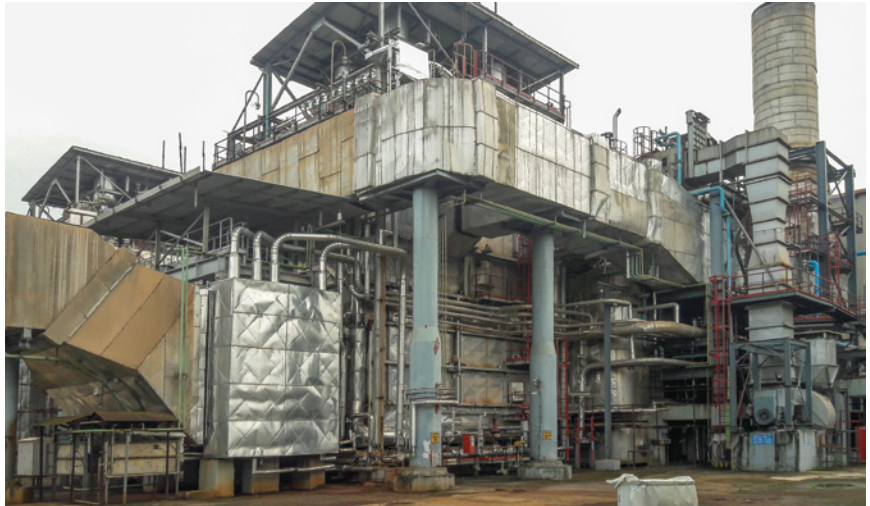
Re-commissioning of HRSG at a petrochemical complex
