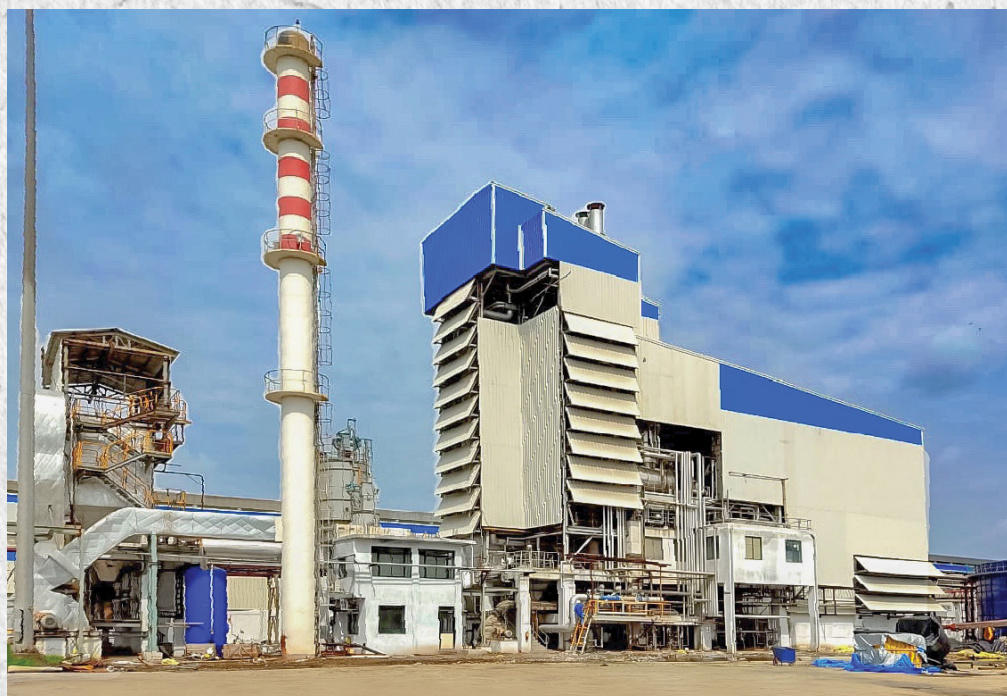
Installation of 100 TPD NRSW fired boiler
