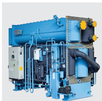
> Thermax's 58 TR hot water driven vapour absorption chiller at an Indian tyre manufacturing plant recovers heat from the air-cooled compressor and utilises it for cooling application in the plant
