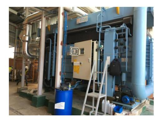
Thermax recently commissioned a 410 TR low temperature hot water driven vapour absorption chiller at the hotel. The chiller is utilising the hot water, as heat source, generated by the natural gas-powered engines. The chiller produces chilled water at 7°C which is used for air conditioning of the hotel.
