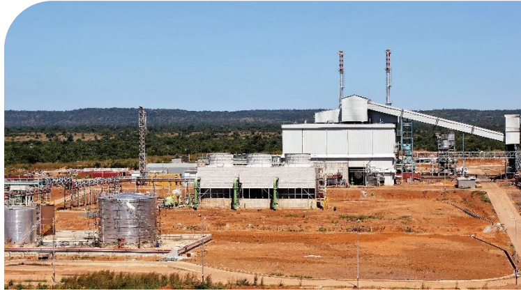
First time synchronisation of 33 MW plant with national grid for an African cement major
