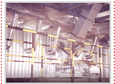
Secondary Over Fire Air Arrangement
