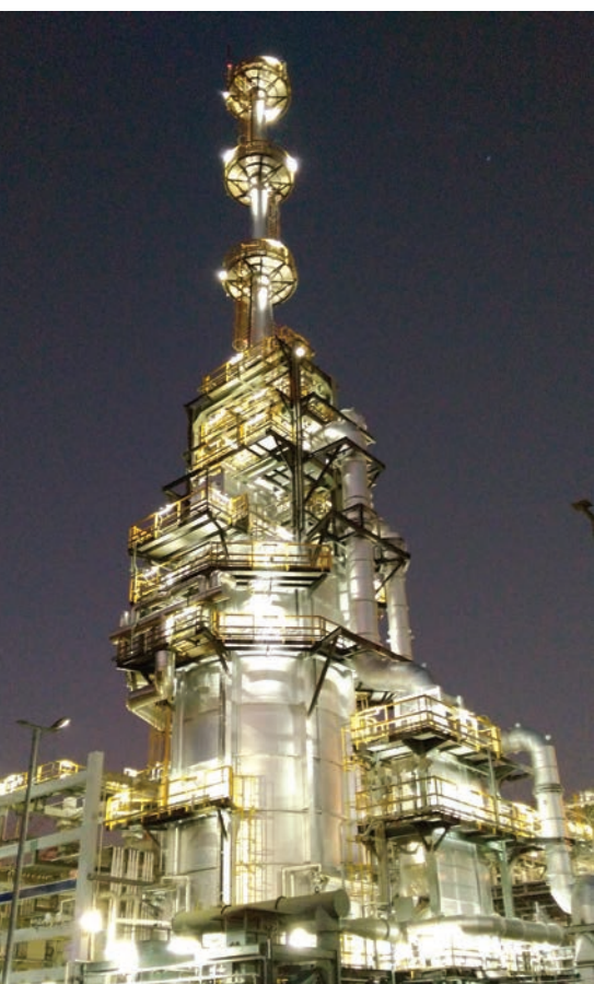
2 units of 6.34 MMKcal/hr hot oil heaters
