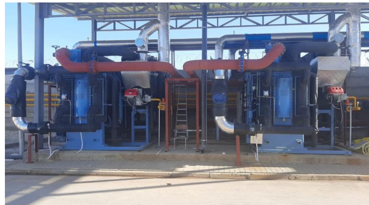
4 gas driven absorption chiller heaters (2 x 410 TR & 2 X 610 TR) for a wiring systems company in Tunisia
