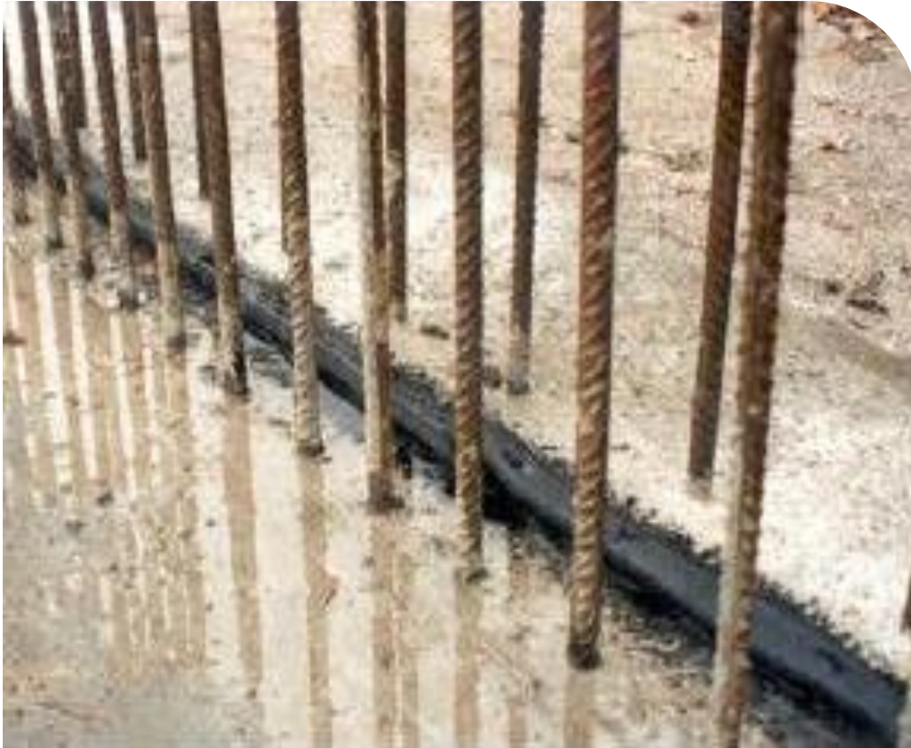
Maxshield@Swellbar - a hydrophilic construction joint water bar and sealant for creating an impenetrable barrier to prevent water ingress in old and new structures
