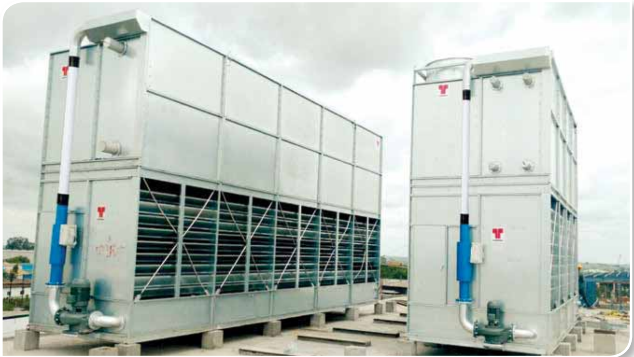
Thermax focuses on the process cooling requirements of industrial firms: two closed circuit cooling towers supplied to a polyfilm manufacturing company in Madhya Pradesh. The equipment helps the client save over 60% in power.
