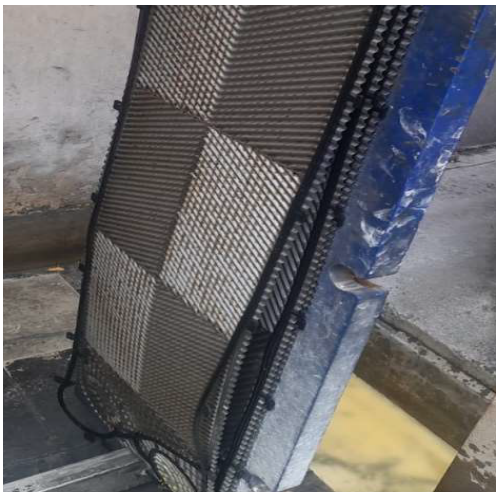
Plate-type Heat Exchanger (PHE) After Treatment
