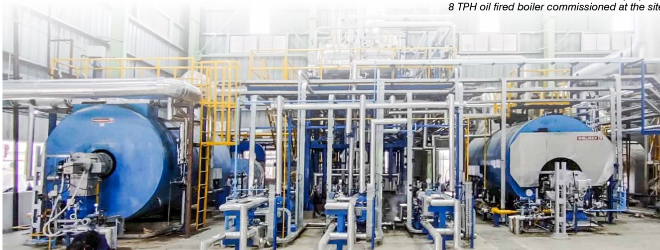
The 3 MnKCal/hr thermal oil heater (left) and 8 TPH oil fired boiler commissioned at the site
