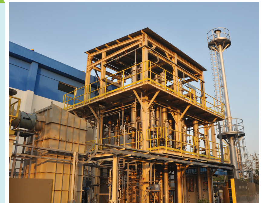
ZLD plant installation at the customer site
