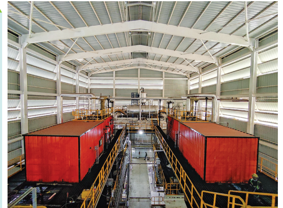
State-of-the-art biomass based boiler plant set up for a leading food major
