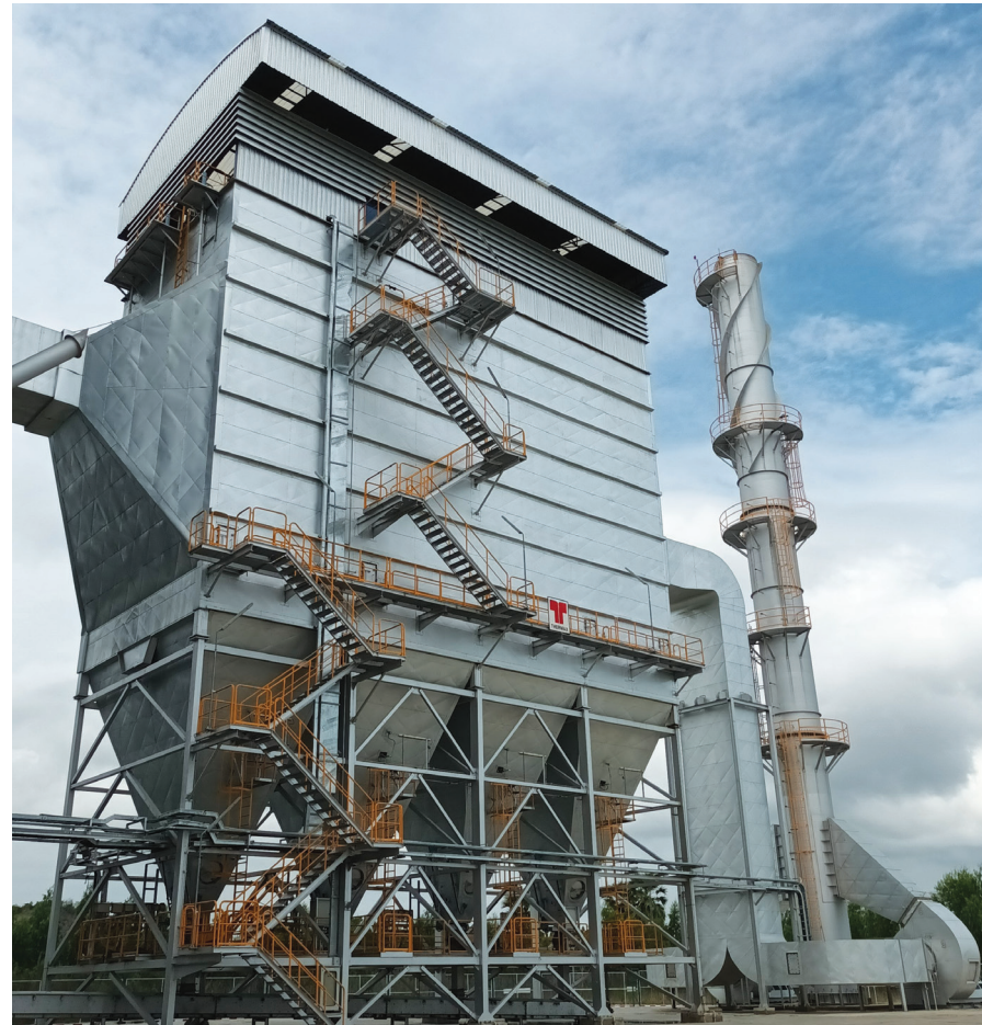
Thermax has installed an electrostatic precipitator (ESP) for a power company in Thailand to control emissions from their 26 MW biomass power plant
