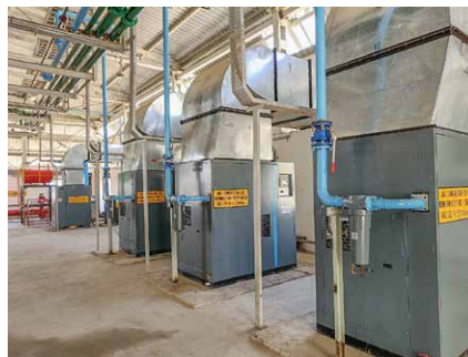
Air compressors and dryers
