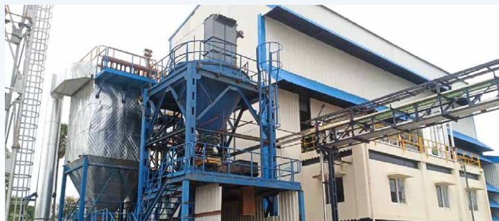
Site image of the 6 TPH reciprocating grate boiler
