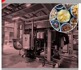
Commissioned a 500 TR vapour absorption chiller at a leading beverages multinational, working in tandem with an evaporative condenser in Chennai, India.
