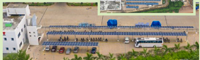
1 MW solar PV installation on the building rooftop and parking lot (below)
