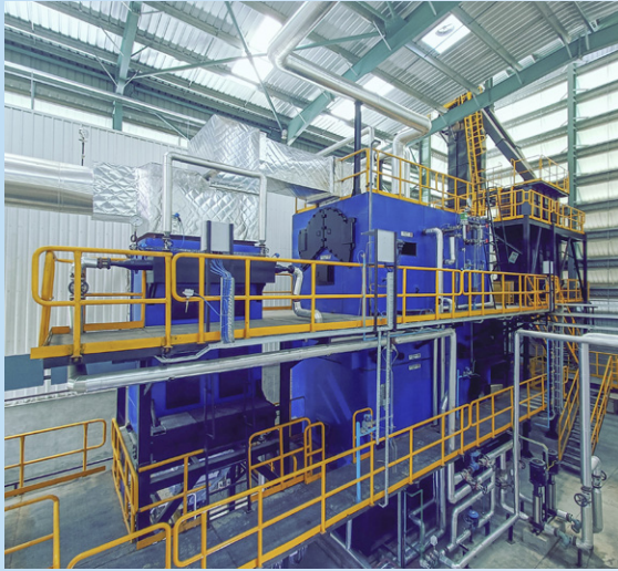
A 10 tonne/hour biomass fired hybrid boiler deployed by TOESL
