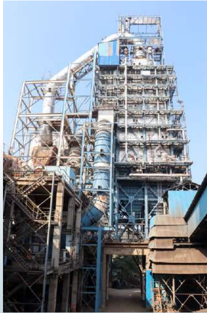
The 30 TPH AQC boiler commissioned at customer site
