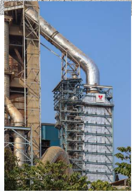
The 19 TPH PH boiler commissioned at customer site
