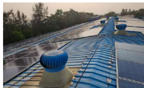
162 kWp solar PV installation at Jhagadia
