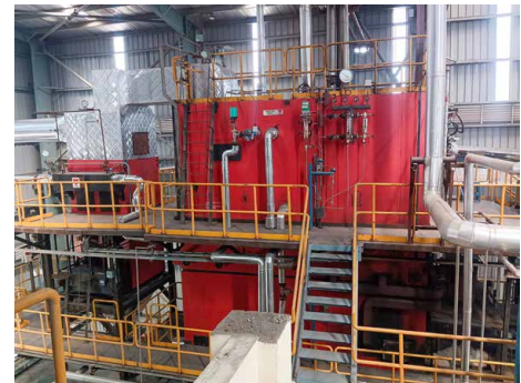
The 8 tonnes/hour biomass fired hybrid boiler supplied at Dahej, Gujarat
