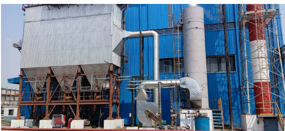
The electrostatic precipitator and scrubber installed at site
