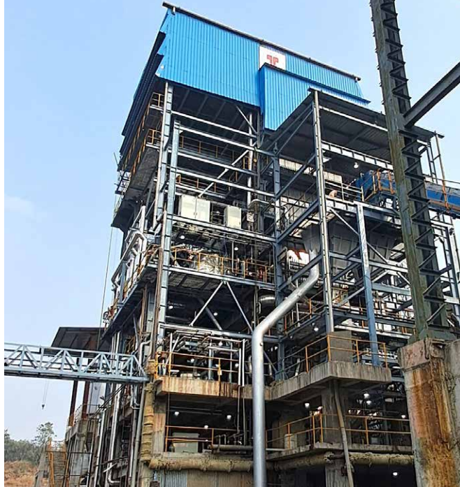
The 32.5 TPH Flexisource™ boiler installed at the paper-based products manufacturer's site at Vapi, Gujarat
