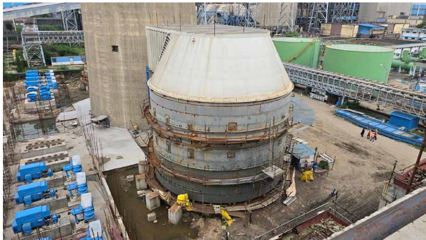
The absorber of the FGD system at the Rihand site in Uttar Pradesh
