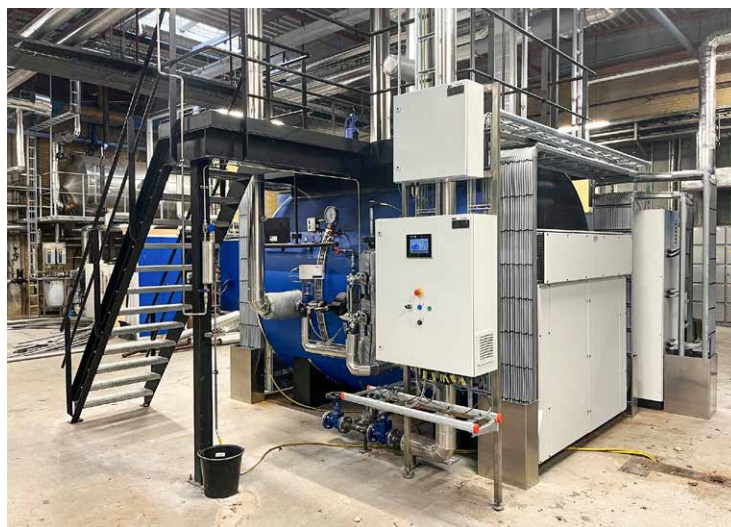
The electric steam boilers installed at Ege Carpets
