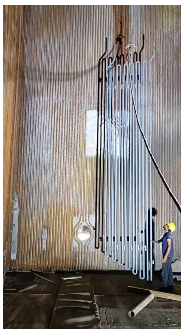
The 170 TPH travelling grate boiler into which the alloy steel superheater coils were replaced
