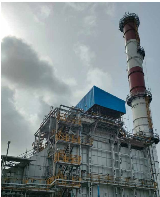
The 125 TPH heat recovery steam generator (HRSG) at West India
