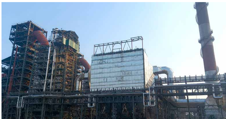
The 2 x 85 TPH sponge iron waste heat recovery boilers at the site in India
