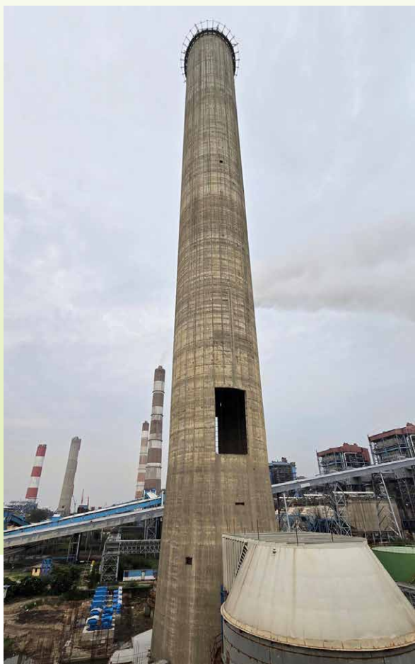
The wet stack of the FGD system at the Rihand site
